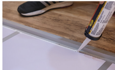
11. Silicone can be used to hold the mirrored panels securely in place
