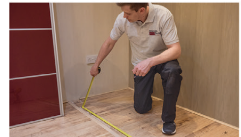
16. Carefully measure the length of track required and make sure the floor is level
