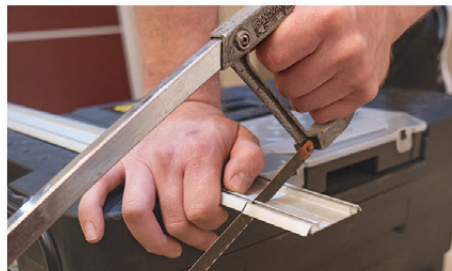
17. Accurately cut the track to size
