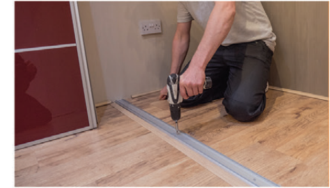
18. Secure the floor track by screwing into the holes provided
