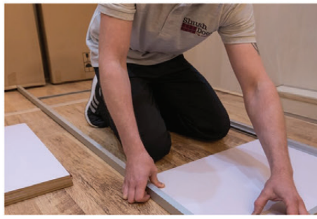
8. Push the bottom panel firmly into the frame
