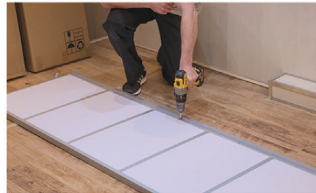
10. Apply the screws to the side rails in order to secure the wooden panels
